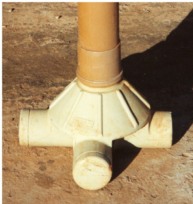
Figure 3.13: Simple plastic junction box used in simplified sewerage instead of expensive manholes.
