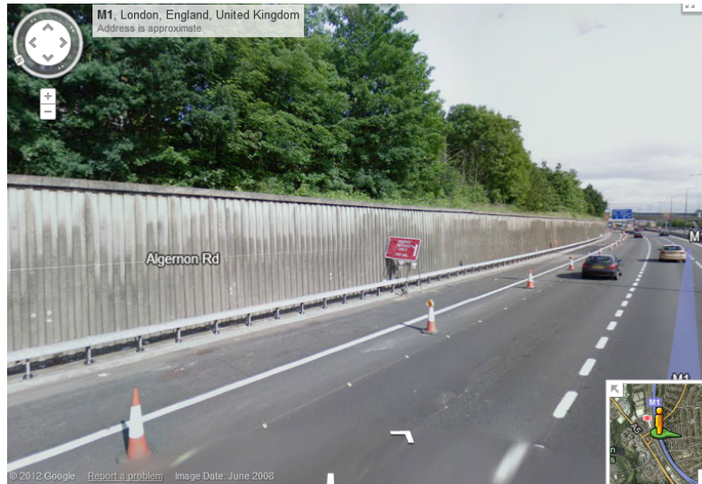
Figure 10.3 Noise barrier along M1 in London, England (Google Street View)
