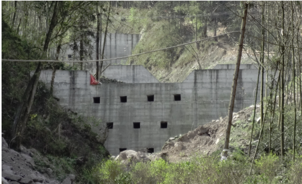
Figure 5.4 Check dam for debris flows
