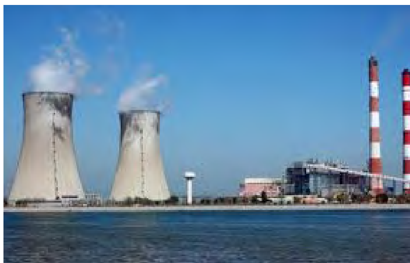
Plate 8.1. Guru Hargobind Thermal Plant, India. Source: http://www.treehugger.com/living/
