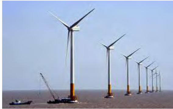
Plate 4.1. Wind turbines at the Donghai Bridge Offshore Wind Farm
