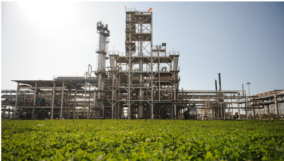
Plate 3.2. Methanol-to-gasoline plant, Shanxi Jincheng Anthracite Mining Group Co. The methanol is made from coal bed methane from an anthracite deposit.
