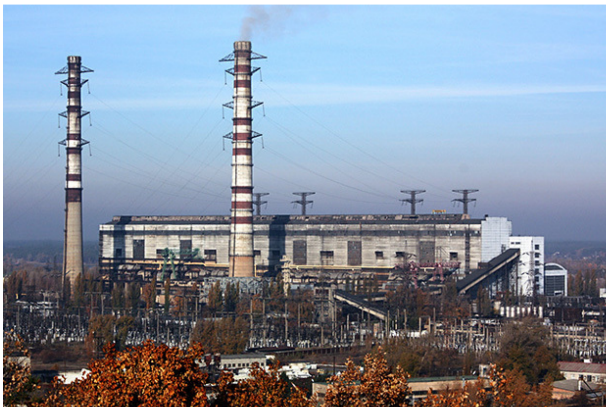
Plate 2.1. Trypilska power station, the Ukraine.
