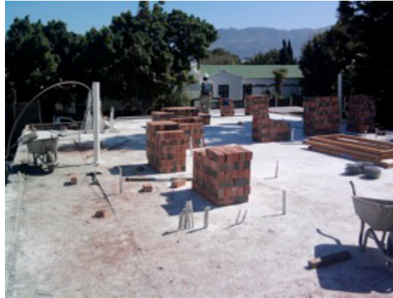
Figure 52: Electrical and Plumbing Installation
