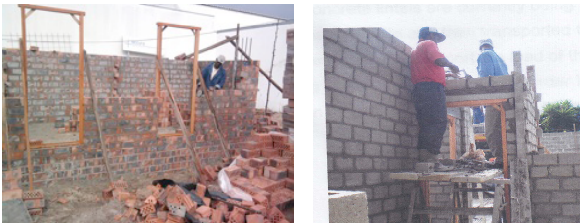
Figure 50: Brickwall and Lintel Construction
