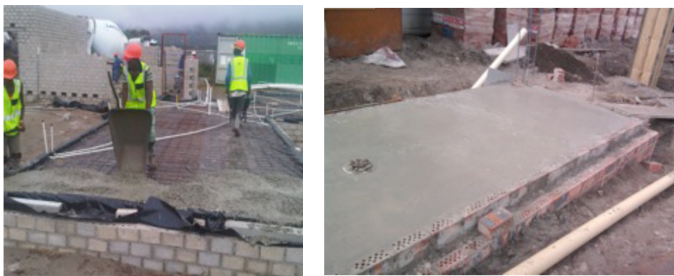
Figure 49: Production of the oversite concrete/surface bed
