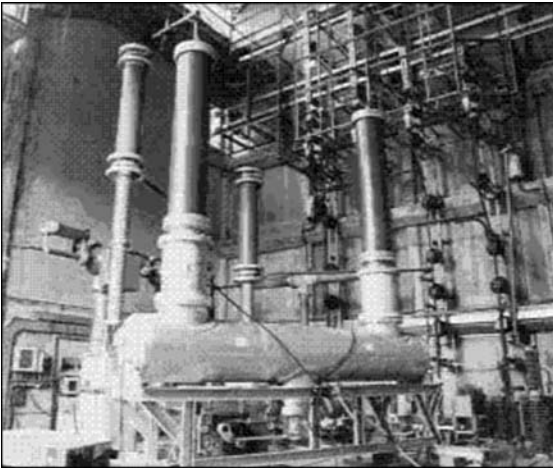
Figure 13 GIS circuit breaker 550 kV 63 kA 50/60 Hz
