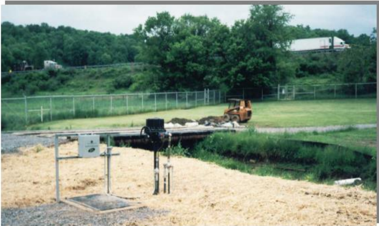
Autonomous Spill Detection Sensor Over Grated Sump Remote Gas Compressor Station, West Virginia
